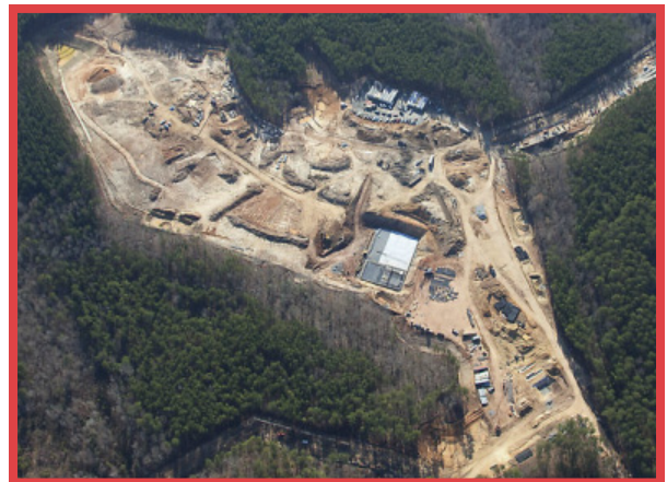
Western Wake Regional Water Reclamation Facility is scheduled to open during the summer of 2014.
