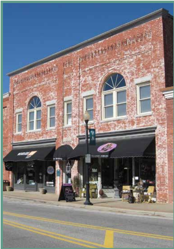
The restored Hinton and Son Hardware building in Apex's Historic Downtown.
