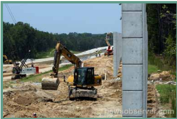
The third leg of the Triangle Expressway from Apex to Holly Springs is currently under construction. (Photo Credit: NewsObserver.com).
