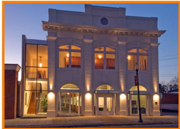
The original Apex Town Hall, built in 1912, was renovated in 2008 and reopened as the Halle Cultural Arts Center.
